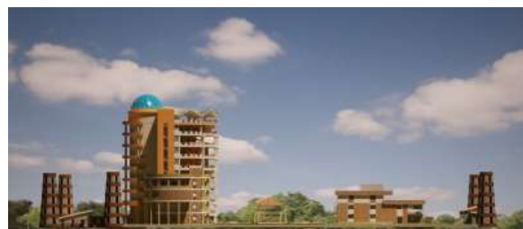
Figure 8. A longitude view of the complex.
