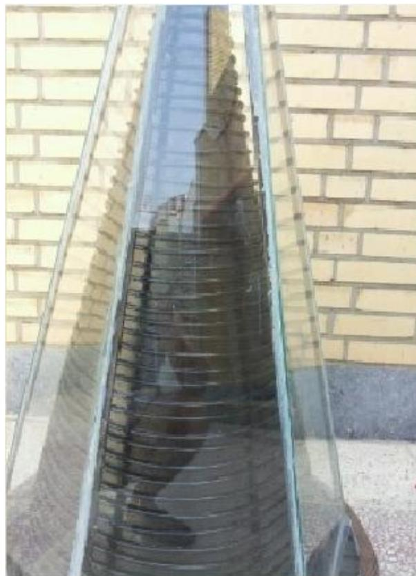
**Figure 2.** Piping and cover install on conical solar collector.
